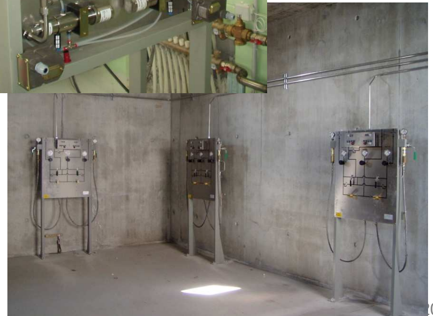
Gas distribution lines: from gas room to underground cavern – CERN (2006)
