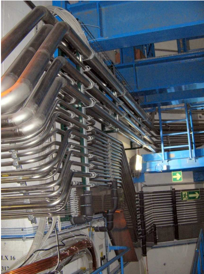
Gas distribution lines: from gas room to underground cavern – CERN (2006)
