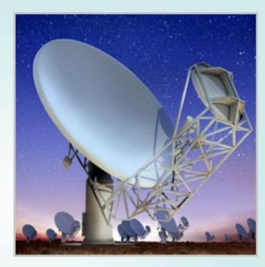
KAT 7: 7 dishes made of fibre glass freq 1.2 - 1.95 GHz max baseline 185 m
